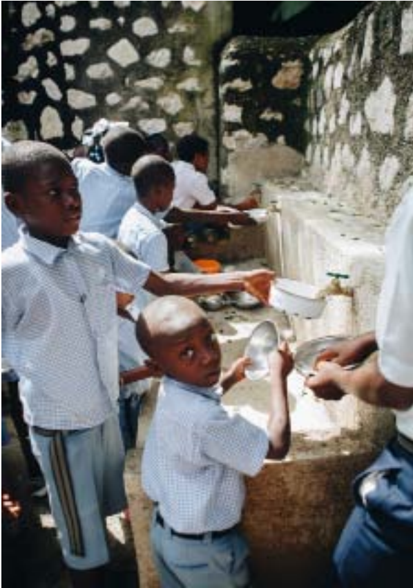
The school sinks in Chauffard utilize clean, gravity-fed water.
