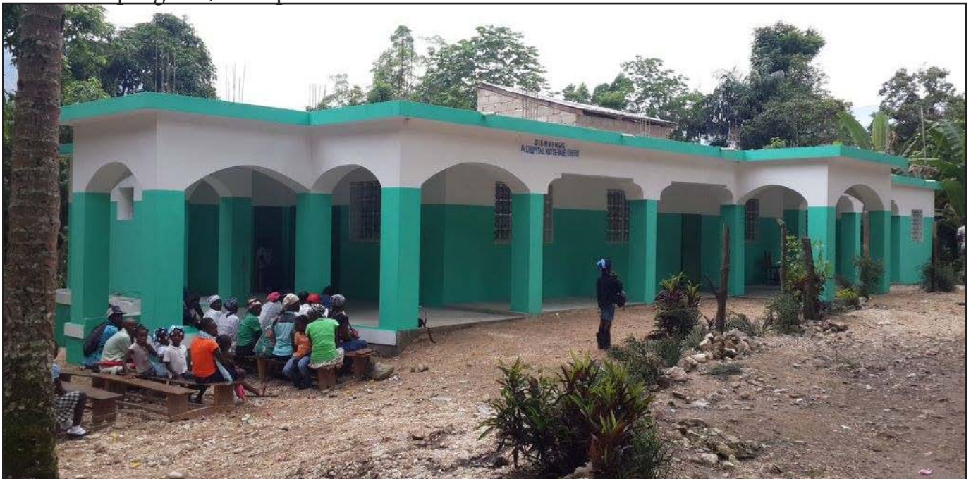
The new health clinic in the village of Chauffard was built with the help of your support! The previous clinic building was 60 years old and damaged in the 2010 earthquake.
